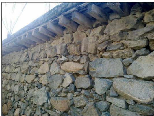
Figure 14. Highlighting Masonry/stone at the exterior
