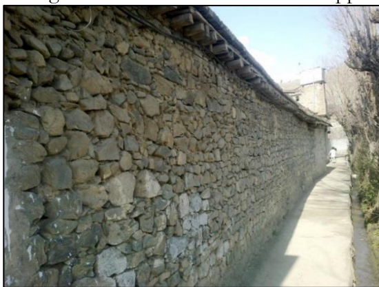
Figure 9 & 10. Showing primary material highlighting the sedimentary stones, and the wood as a structural element.
