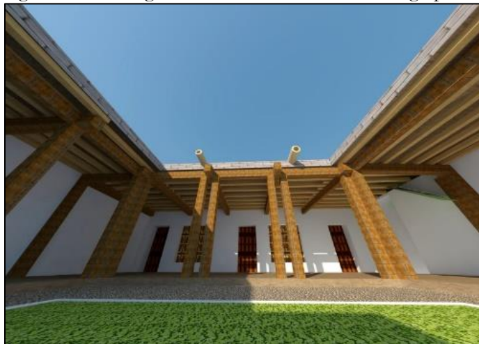
Figure 24. Pic showing the parnalas/rainwater drains from the roof
