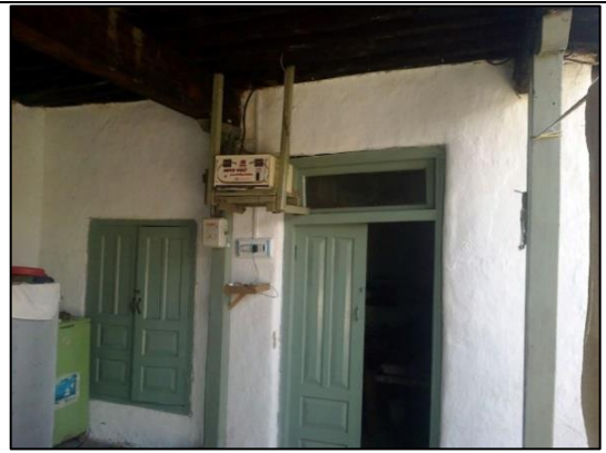
Figure 15. Highlighting mud/cladding on the interior
