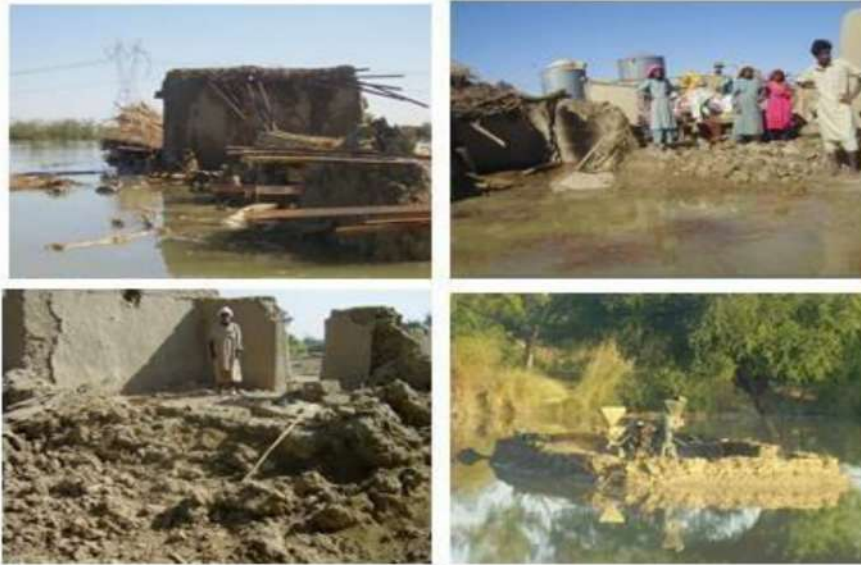
Figure 2. Clay house and prominent damage (Source: RCDS)
