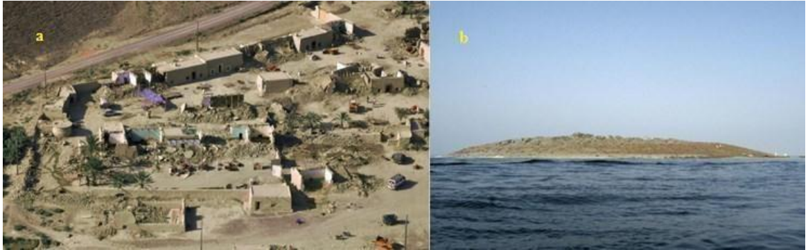
Figure 3. 2013 Earthquake in MW 7.7 Awaran. (a) An aerial view of the Oran area's destruction. (b) A view of the island following an earthquake in Awaran [8]
