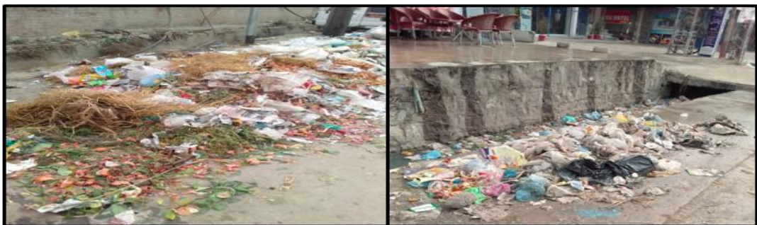
Figure 9: Garbage Heaps at Roadside
