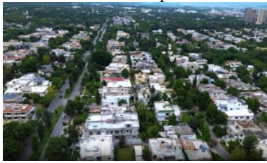
Figure 5. Rooftops View of ISB [37]
